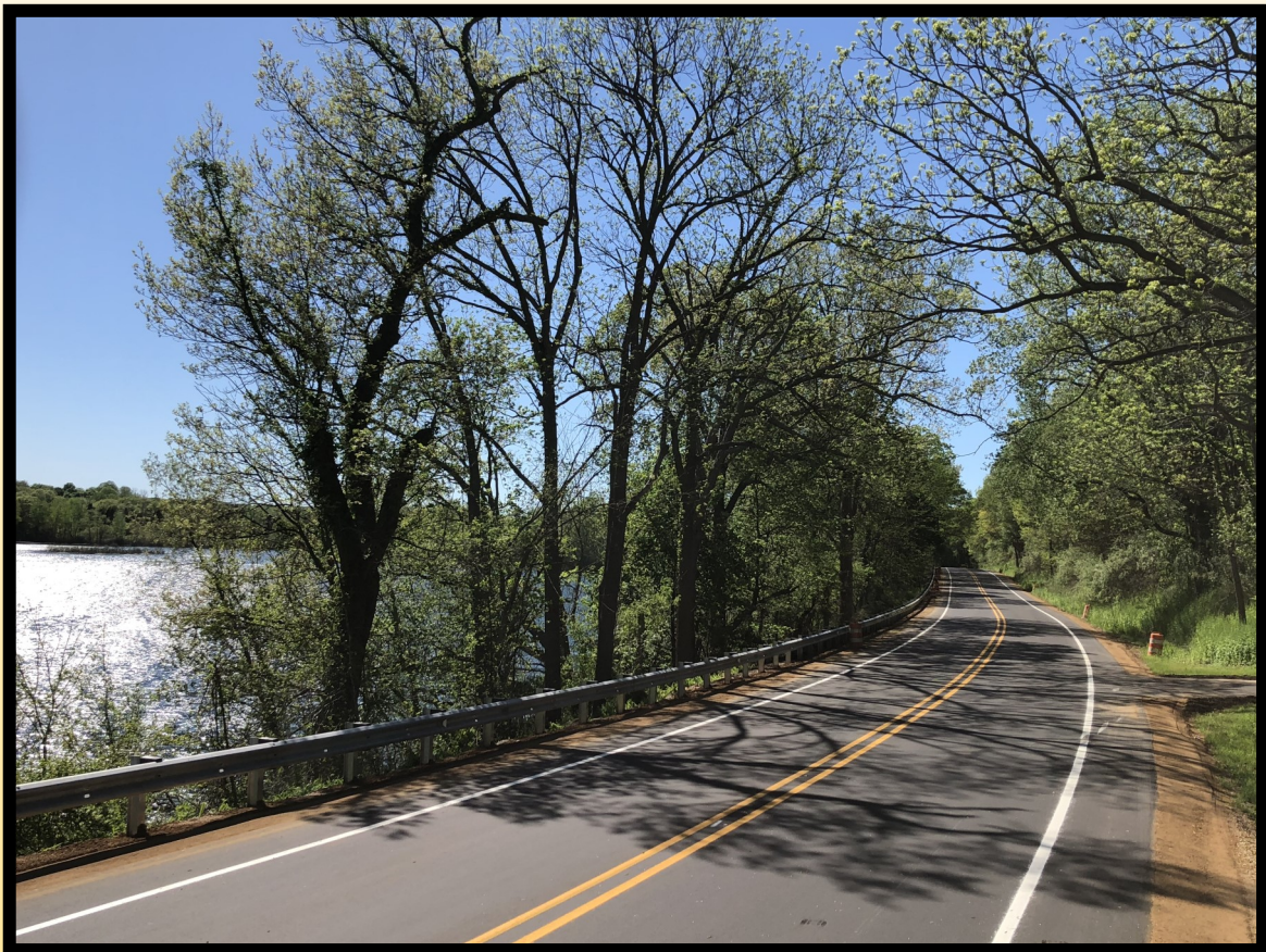
Ravine Road—12th Street to US-131 Alamo Township
