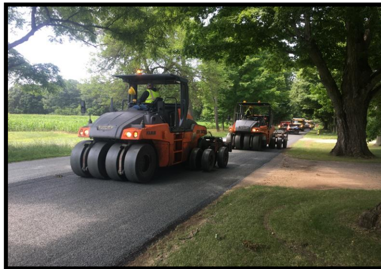
KL Avenue - 4th Street and 8th Street, Oshtemo Township
