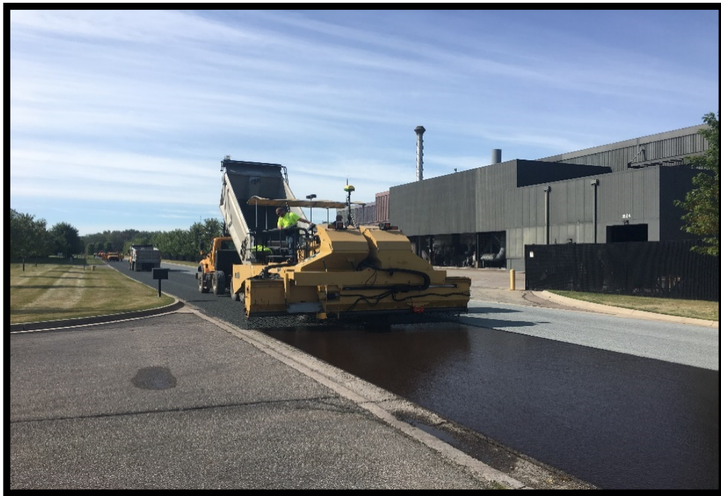
Park Circle Drive - Sprinkle Road to Cork Street Comstock Township
